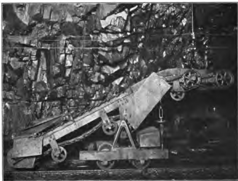
PORTABLE LOADER, INSTALLED TO FACILITATE THE LOADING AND DISPOSAL OF ROCK
